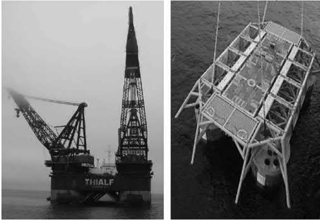
Figure 19-30 Installation of Temple Using THIALF in the Ormen Lange Field [33].
