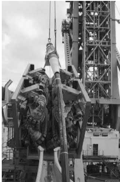
Figure 30-24 Lifting of a Flexible Jumper from a Barge.
