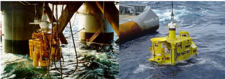
Figure 24-29 Tree Installation by Drill Pipe (Left) and Rig Winch (Right).
