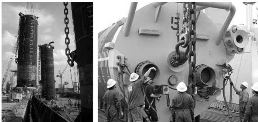
Figure 4-6 Suction Pile [10].
