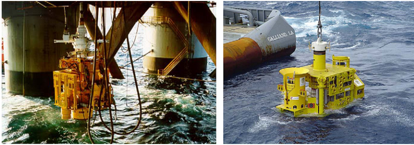
Figure 22-42 Tree Installation by Drill Pipe (Left) and Rig Winch (Right)
