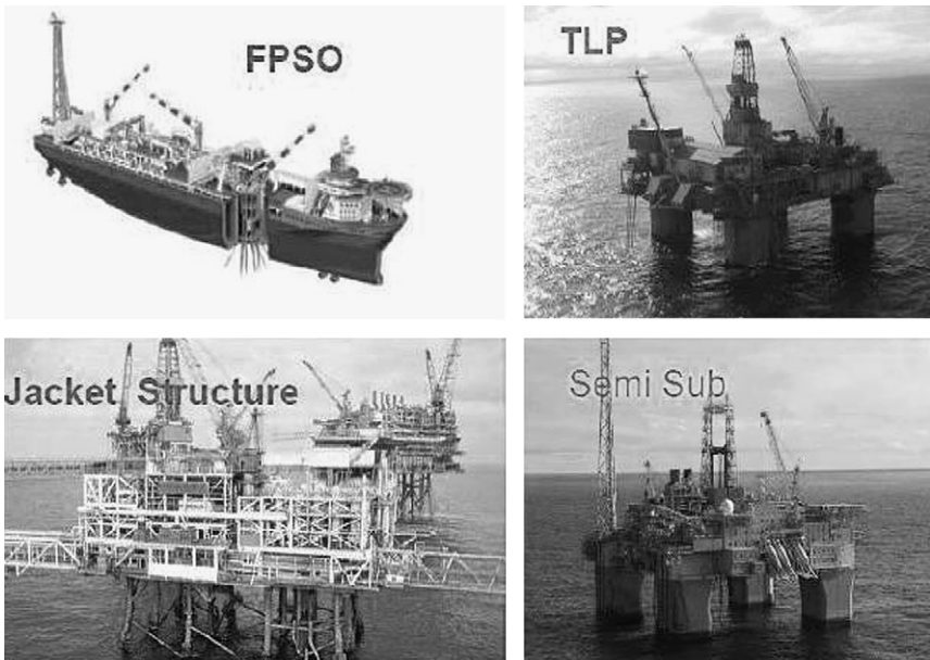
Figure 2-13 Typical Host Facilities [5]
