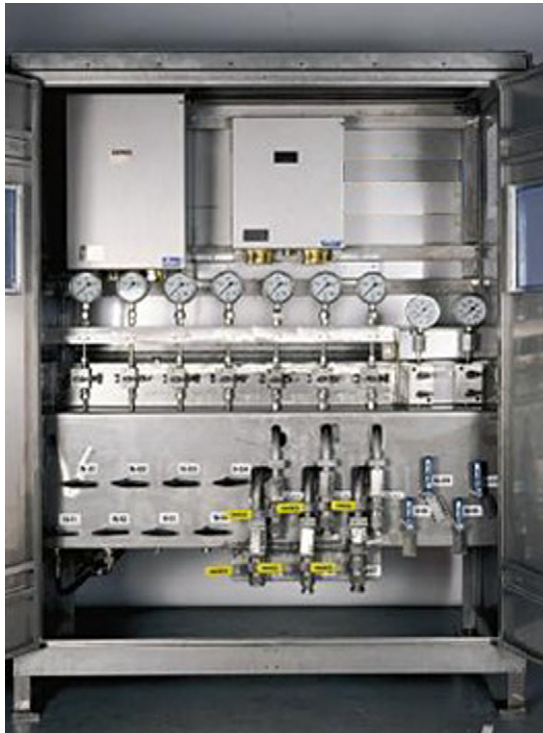
Figure 3-2 Topside Umbilical Termination Assembly (TUTA) [1]
