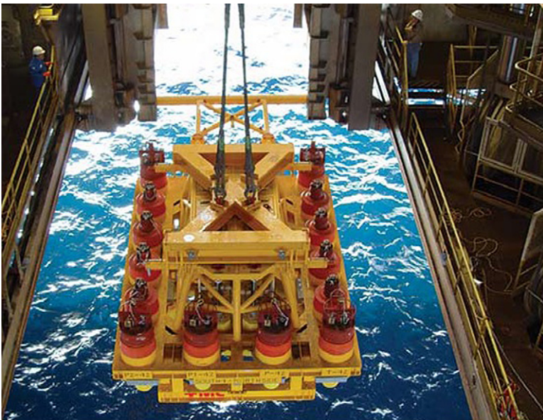
Figure 6-13 Subsea Manifold [8]
