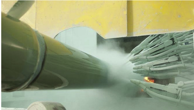
Figure 24.3 Fusion-bonded epoxy powder application onto heated pipe [9].
