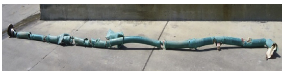
Figure 27.7 Example of failure of reinforced thermoplastic pipe line due to excessive loading at couplings.
