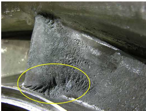
Fig. J.43 This design exhibits more damage at the hub than at the shroud intersection. This counter intuitive behaviour is a feature of certain hydraulic designs and can be associated with low flow operation.
