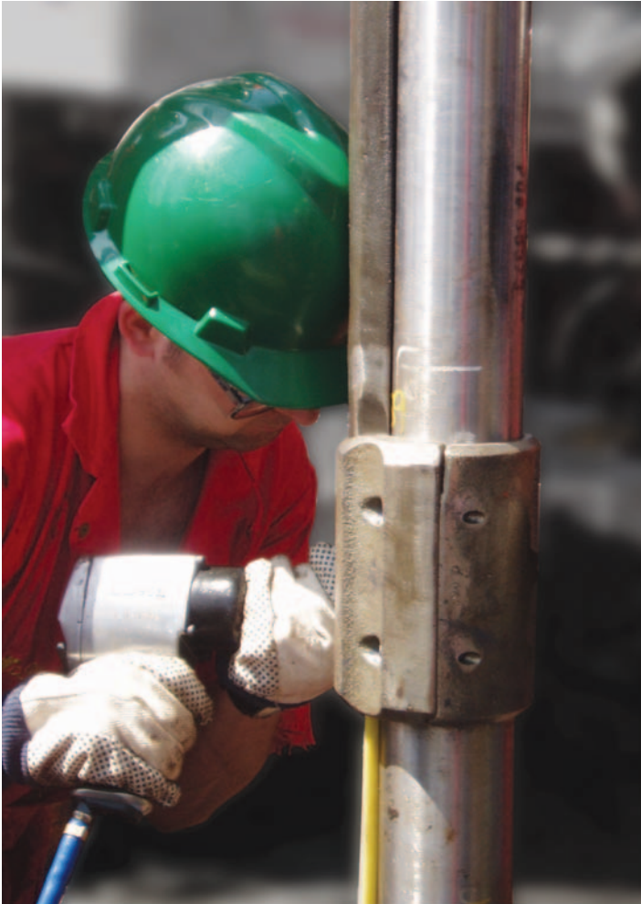
Figure 12.16 Installing a control line protection plate.
