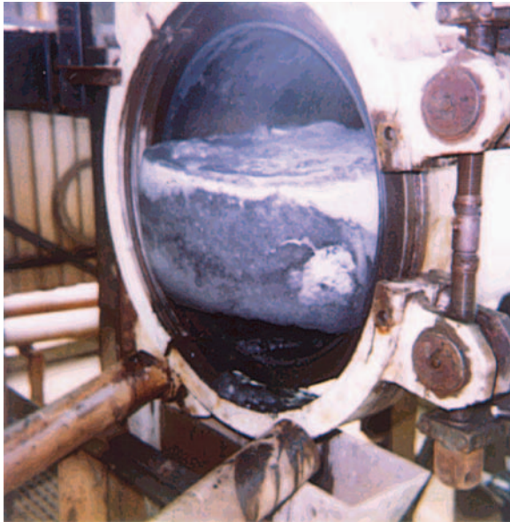
Figure 7.24 Hydrates in a pig receiver.
