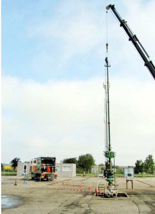
Figure 9.1 Slickline on location in the Netherlands. Photograph courtesy of Bob Baister.
