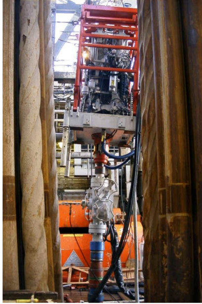
Figure 10.44 Properly support and secure the injector head throughout the operation!
