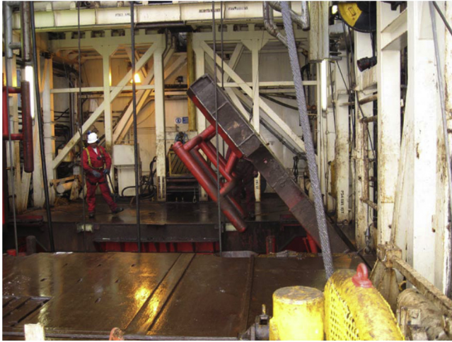
Figure 15.4 Opening the moonpool doors on the Helix Seawell. Photograph courtesy of Helix Well Ops.
