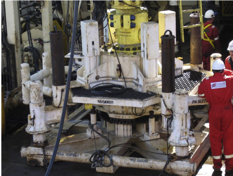
Figure 15.12 The tree running tool being made up to the lubricator.
